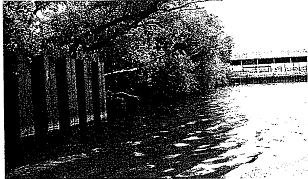
Mixture of sheet pile bank and overhanging vegetation in the SBCR
